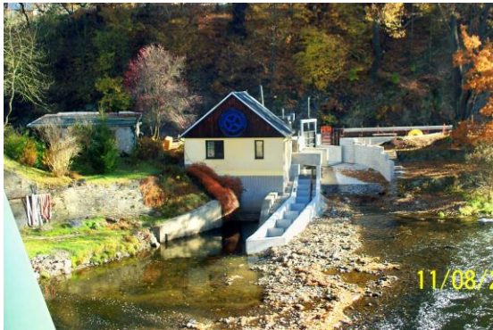
Water power station for Rolle mill with fish stair
