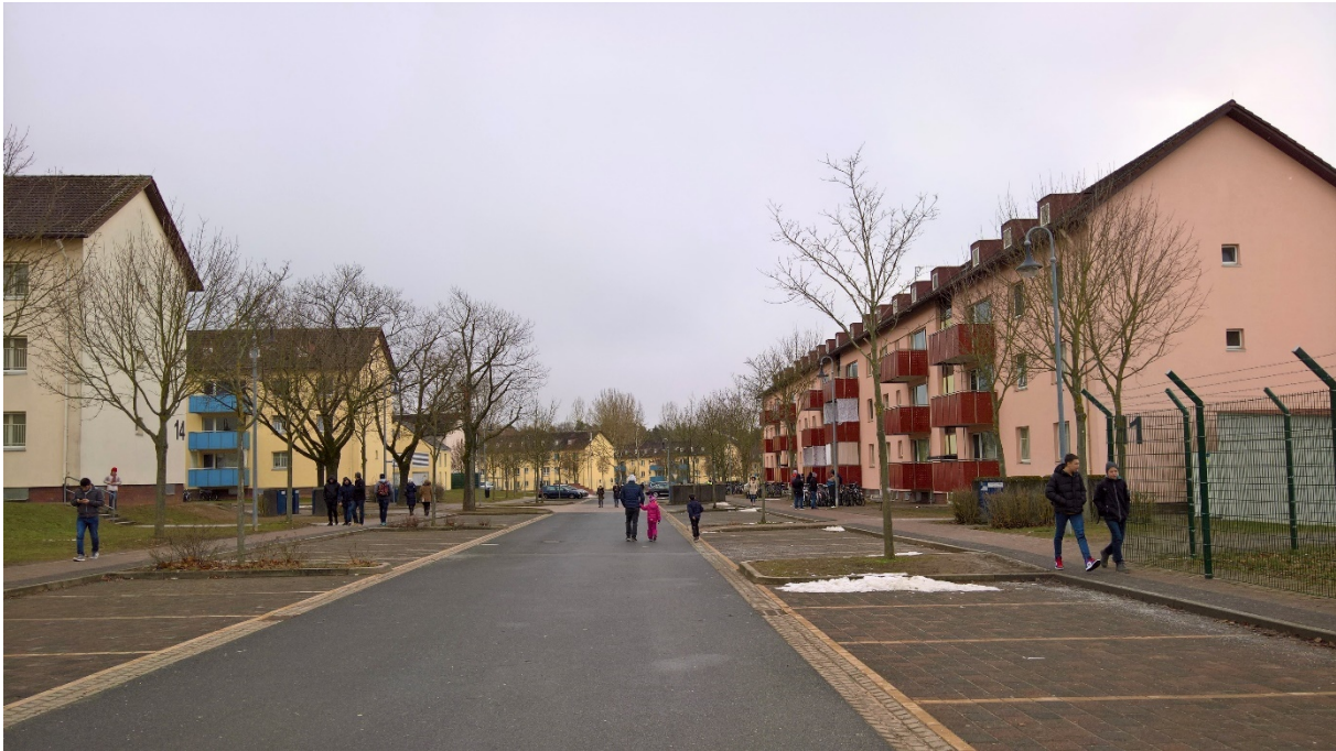
Figure 4: Walkways on the territory of the Initial Reception Facility AEO Bamberg
