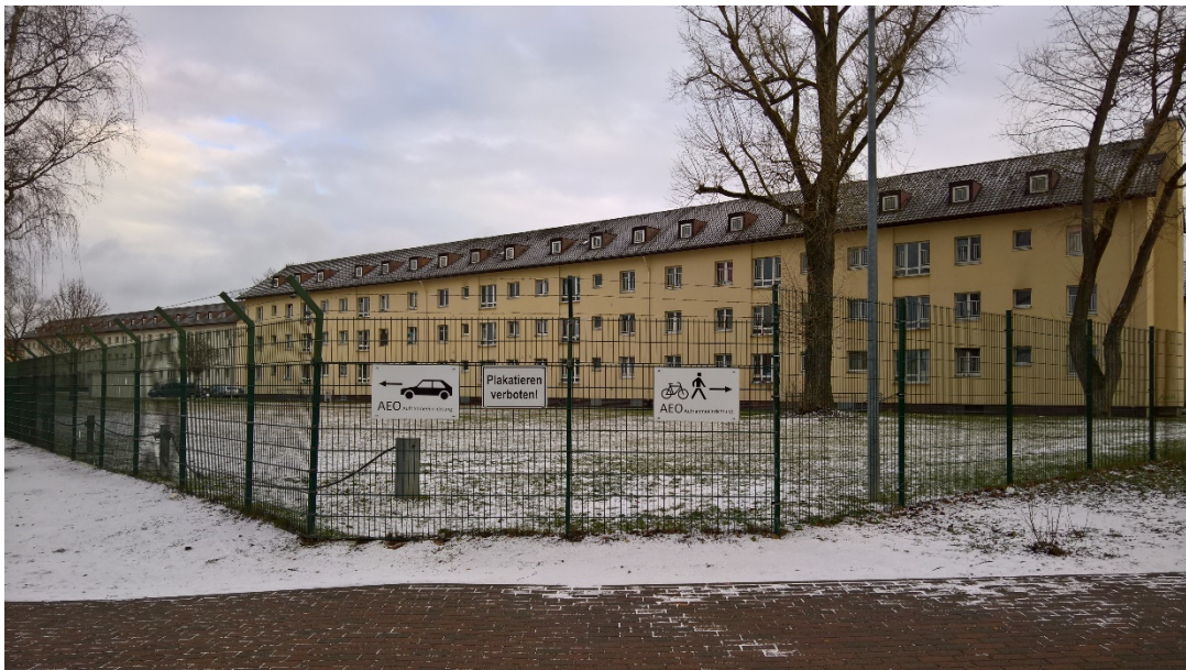
Figure 3: Initial Reception Facility AEO Bamberg, Germany, entrance directory
