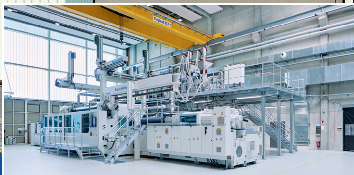
New Research Centre of the Federal Cluster of Excellence MERGE in Chemnitz
